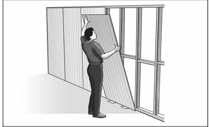
FIGURE 4 SHEET INSTALLATION
